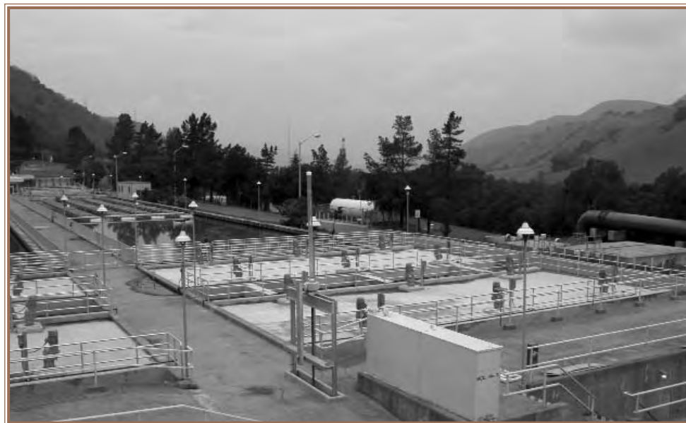
Sunol Valley Water Treatment Plant
