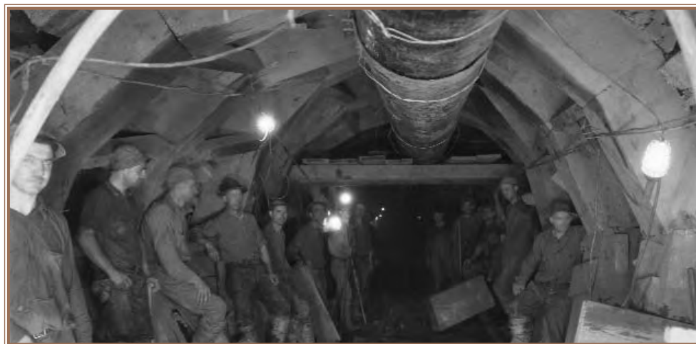
Construction workers in Coast Range Tunnel 1930
