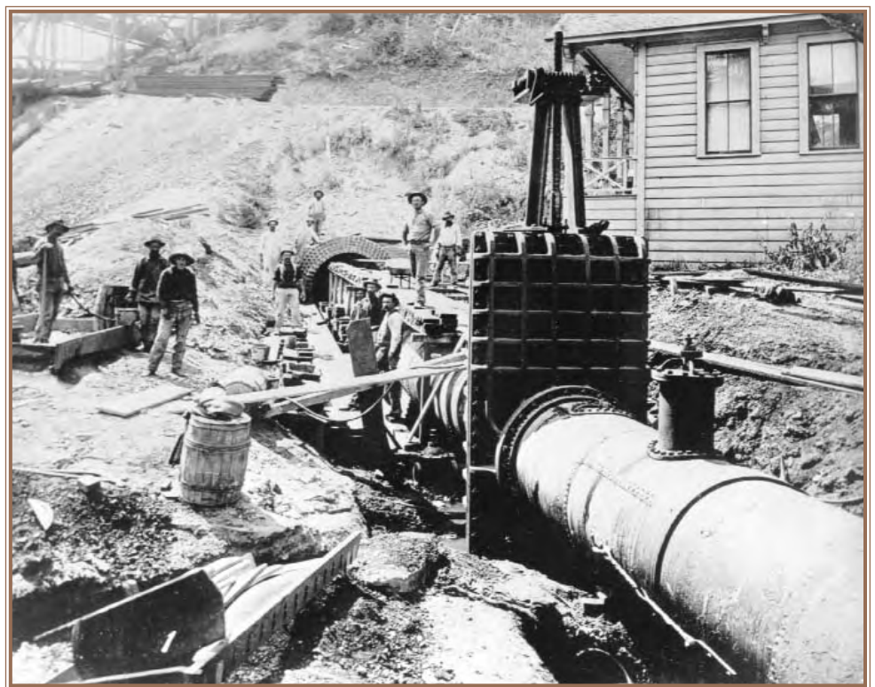
Lower Crystal Springs Dam outlet works under construction 1888
