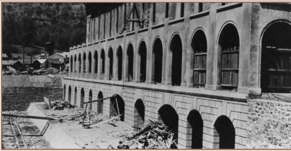
Old Moccasin Powerhouse under construction 1924
