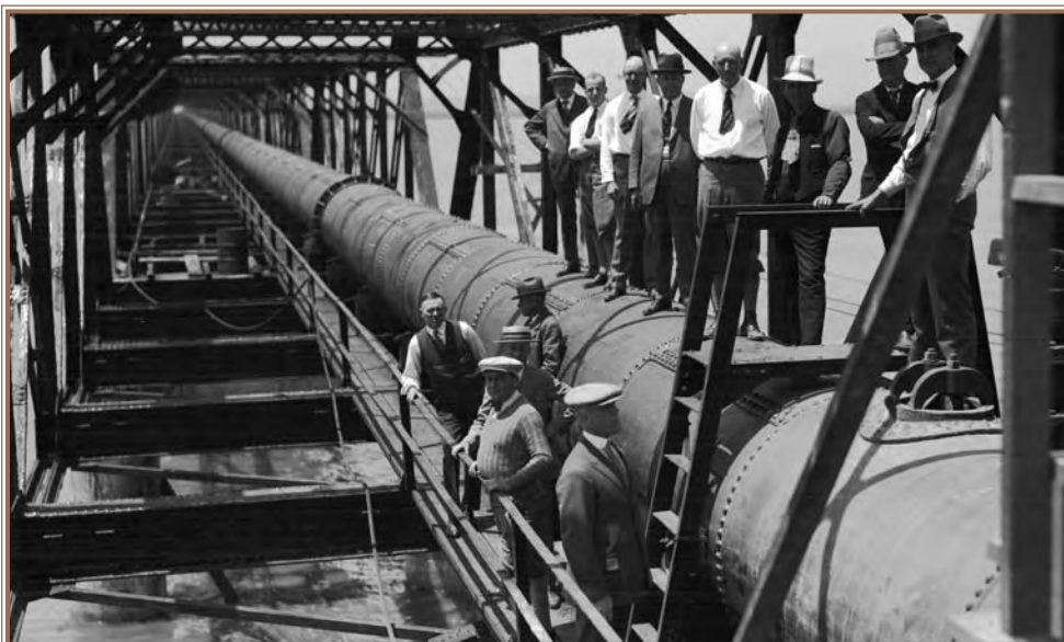
Bay Division Pipeline No. 1 on Trestle Bridge 1925
