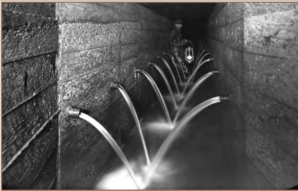
Sunol Filter Galleries 1906
