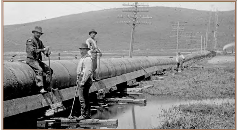
Crystal Springs Pipeline No. 1 after earthquake 1906
