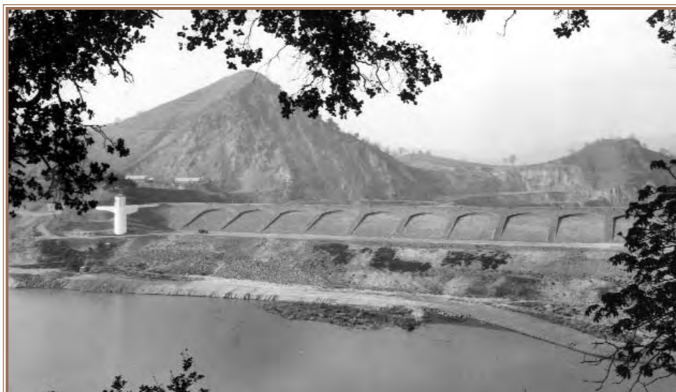
Calaveras Dam and outlet tower 1926
