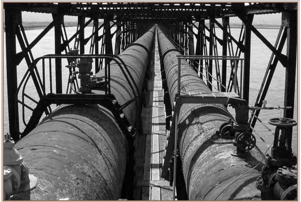
Bay Division Pipelines on trestle bridge
