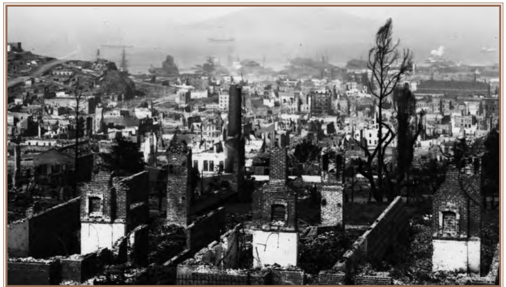
Aftermath of Great Earthquake and Fire 1906
