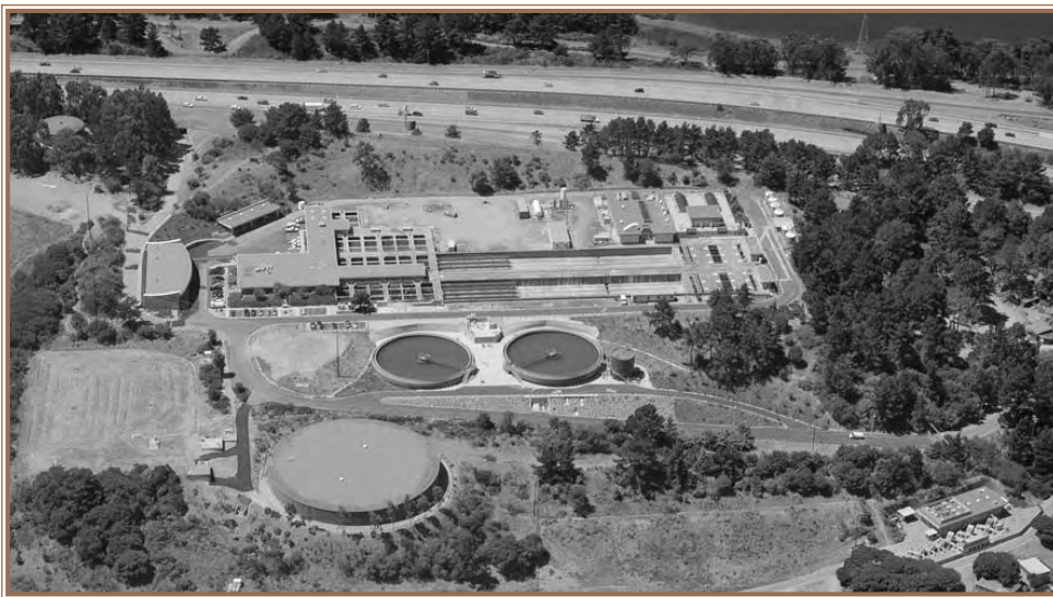
Harry W. Tracy Water Treatment Plant aerial view
