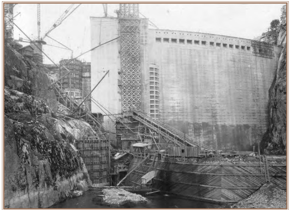
O'Shaughnessy Dam, upstream face 1923
