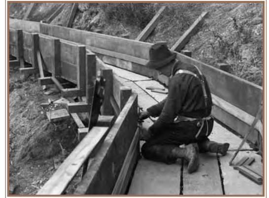
Construction of Stone Dam Flume 1871
