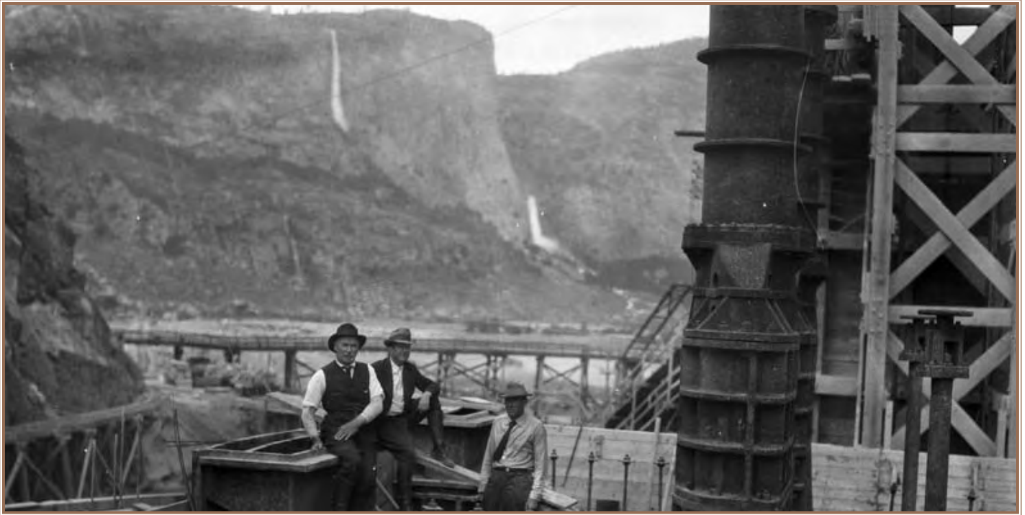
Construction at O'Shaughnessy Dam (Michael O'Shaughnessy at far left) 1922
